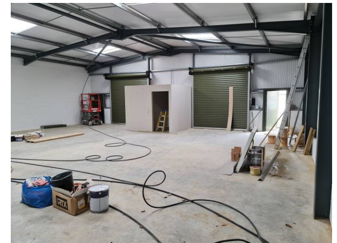
Photo during the construction period.
